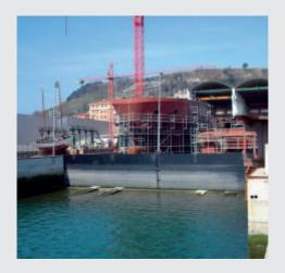
A major step has been achieved by upgrading and lengthening the slipways. The two slipways for new constructions have been given a 60 m long side wall and two front gates. As a result, the shipyard is able to build vessels up to 85 m length and, if necessary, with up to 30 m beams. The side wall will also be used as support for a gantry crane which will be able to handle blocks directly over the slipways for future projects.
